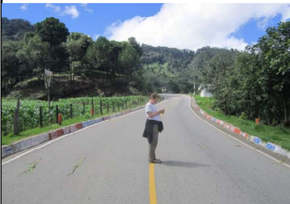
Taking GPS location of the road crossing where the pipe from the existing lower spring location joins the main distribution line (right just off the road)
