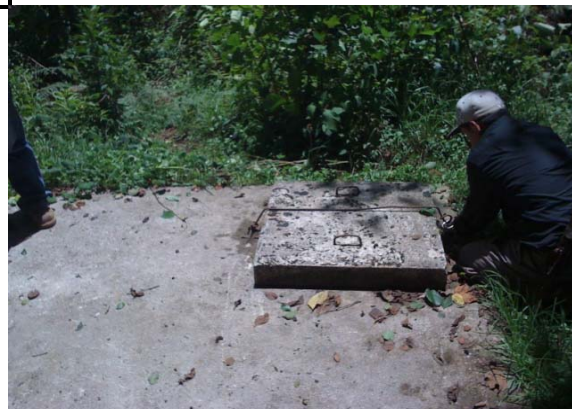
Existing 20,000L tank
