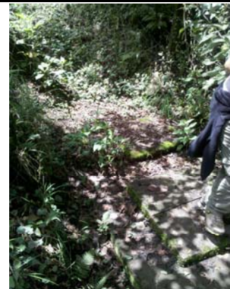
Pressure break box in the lower portion of the water distribution system.
