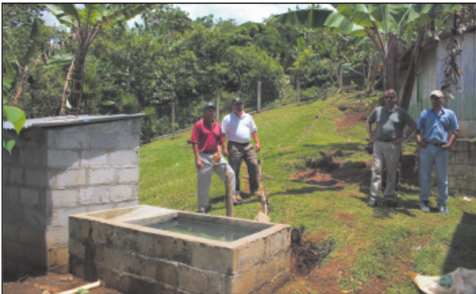
FWA volunteers survey a pila, or clothes washing station, that was built as part of the 2007 water and sanitation project in El Ponciano, Honduras.
