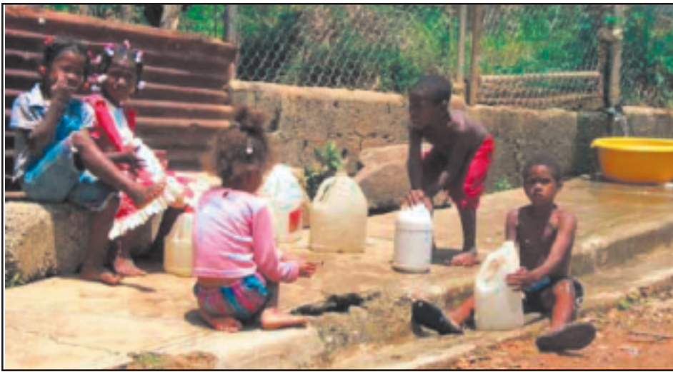
Children of Miramar collecting water from the street and sidewalk that has leaked from the municipal storage tank.
